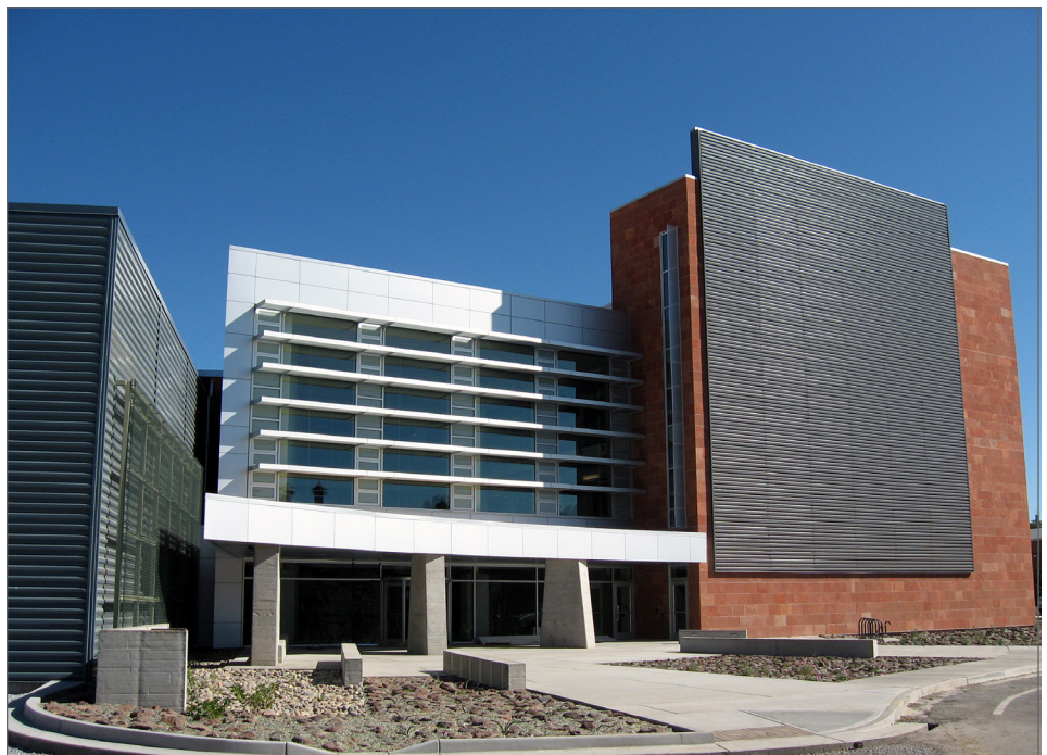
Solar air heating system at the Northern Arizona University
